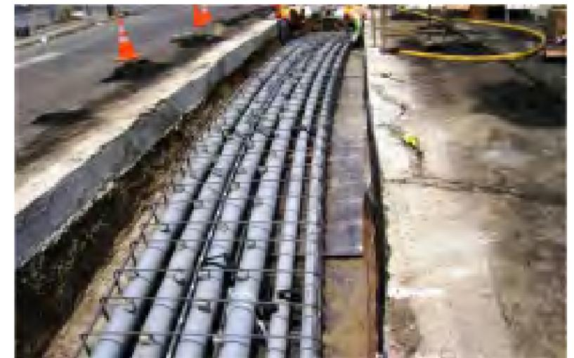
Figure 2: Installation of Duct Banks during Streetscape Construction
